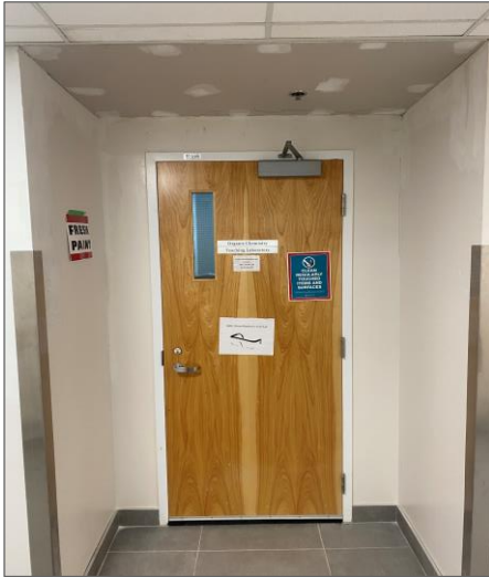
Photo 11 – South door to Room E316 where new drywall has been implemented.
