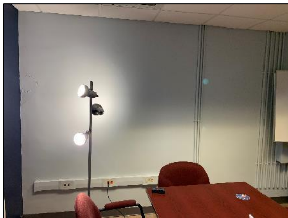
Photo 2 - View of south wall.
